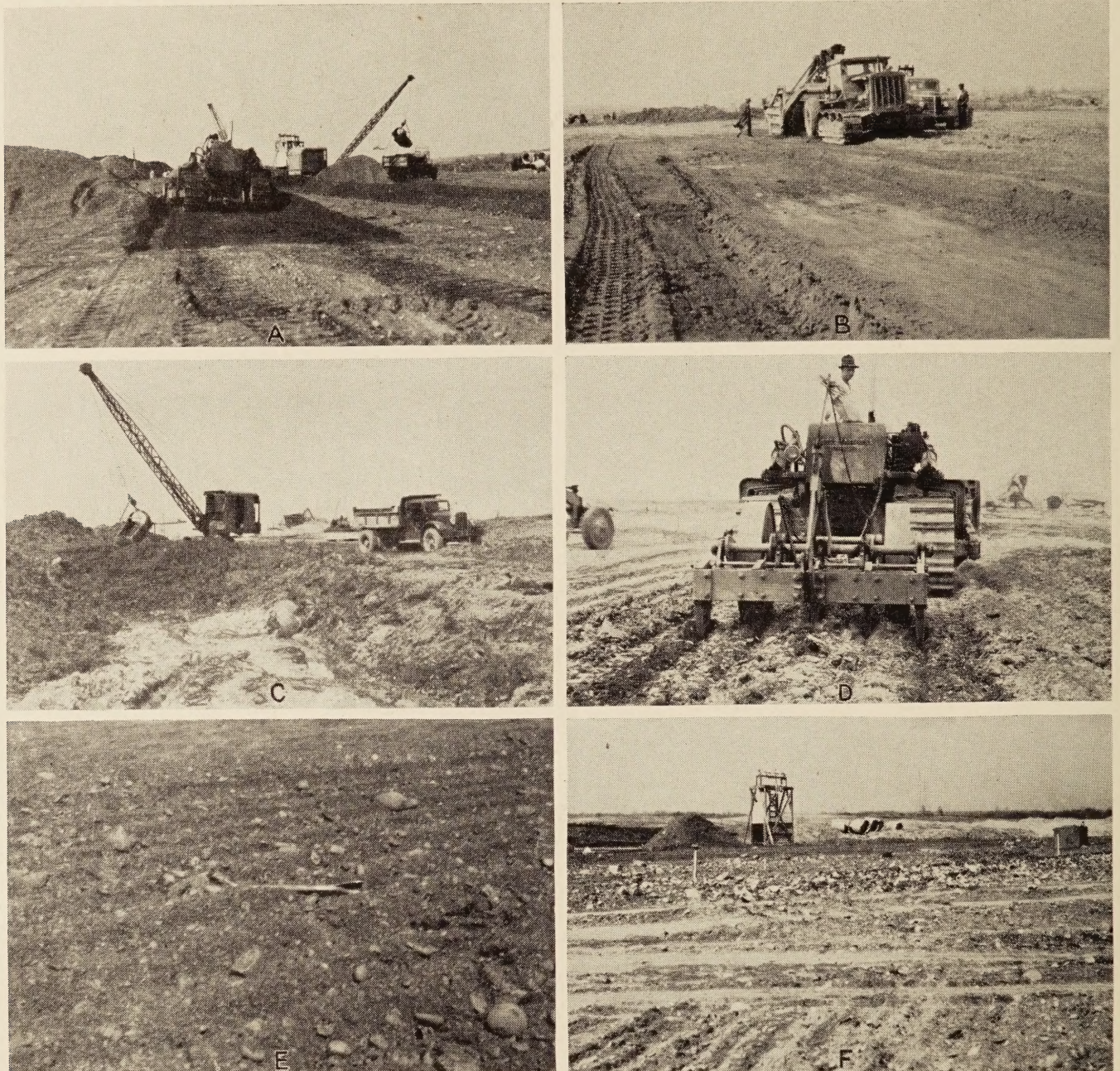
FIGURE 8.—CONSTRUCTION OF RUNWAYS: A, GRADING OPERATIONS; B, THIN LAYERS OF MUCK BEING EXCAVATED BY SCRAPER; C, DEEP MUCK BED BEING EXCAVATED BY DRAGLINE; D, SCARIFYING MATERIAL WITH HEAVY-DUTY ROOTER; E, OVERSIZE STONE BROUGHT TO SURFACE BY SCARIFYING; AND F, OVERSIZE STONE IN EXCESSIVE AMOUNTS GENERALLY ENCOUNTERED AT RUNWAY INTERSECTIONS.
